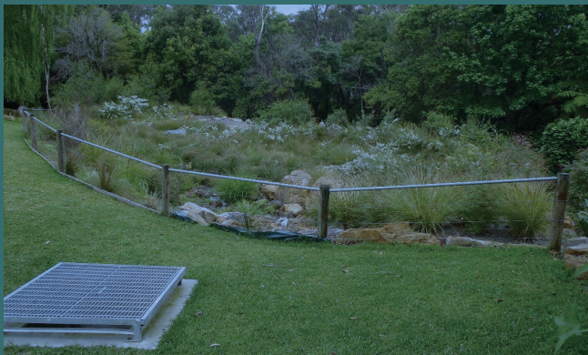
Margaret Ave, Hornsby Heights – Large end-of-pipe biofilter
