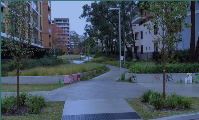
Orara Park, Waitara – Biofilter and stormwater harvesting (for irrigation of Mark Taylor Oval)
