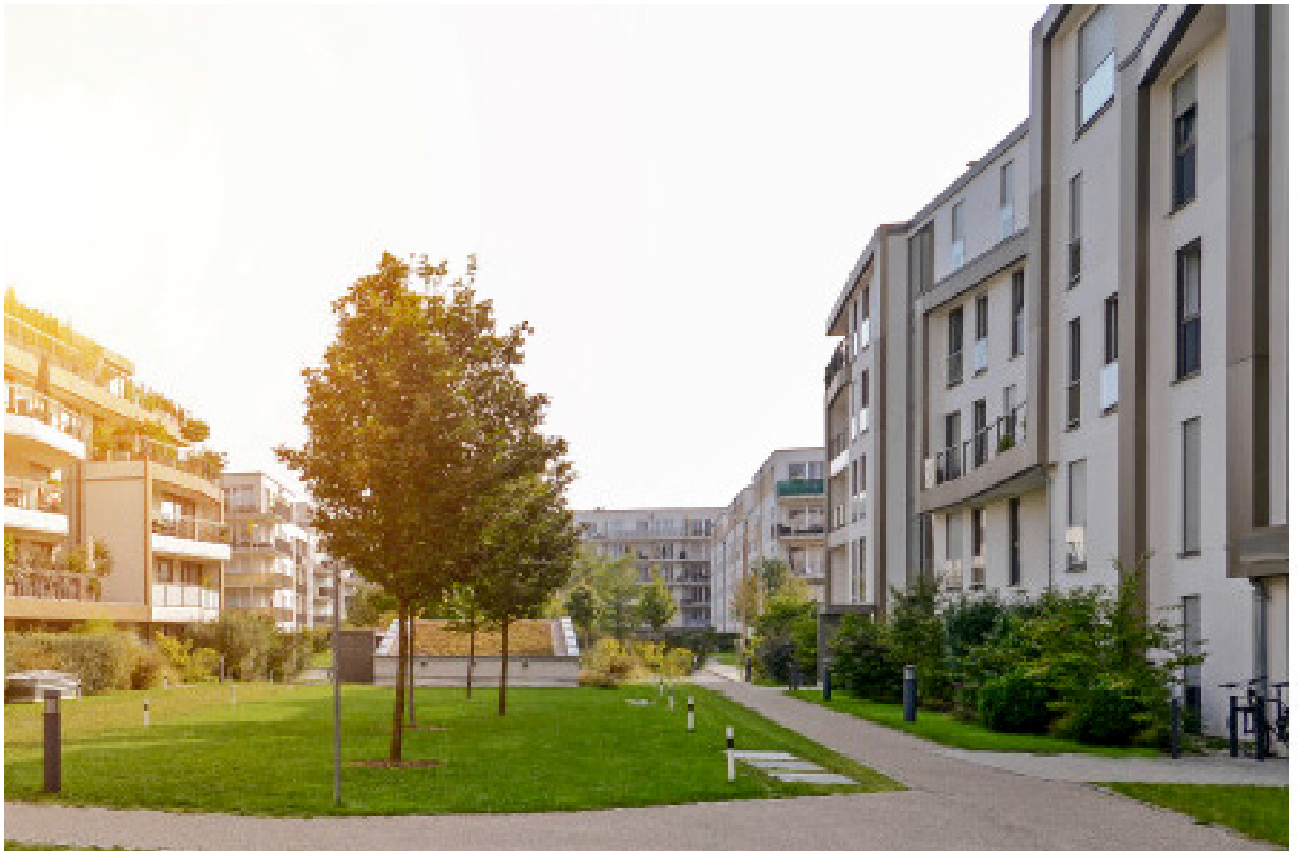
Photo 3 – Sustainable Design (eg stormwater harvesting and green roof)
