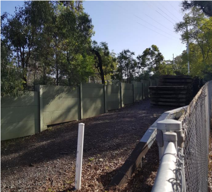
Figure 33 - A2-6 Trees - Looking North along corridor at TfNSW driveway between Chapman Avenue and Beecroft Station
