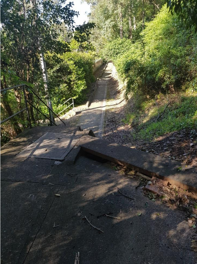
Figure 42 - A4-4 Existing Retaining Structure – retaining wall along existing stair corridor looking south along the stair path towards Binomea Place from Hampden Road
