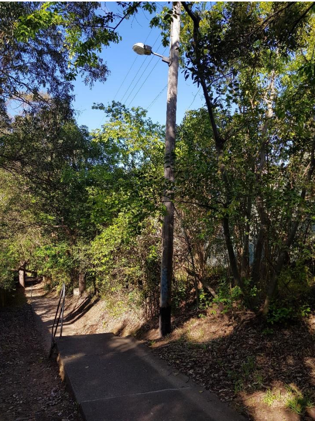
Figure 39 - A4-2 Existing Lighting – Looking south along the stair path towards Binomea Place from Hampden Road
