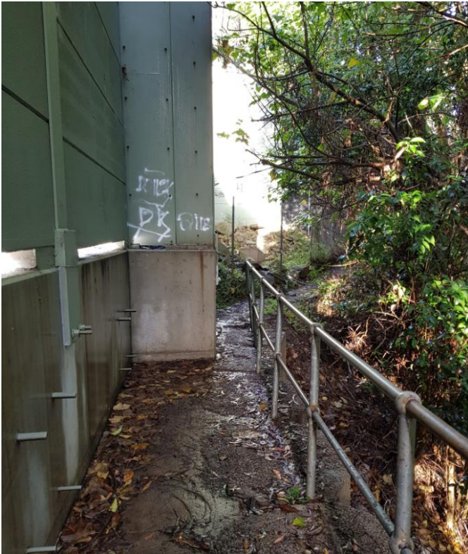
Figure 19 – Byles Creek Crossing - Looking south along existing noisewall
