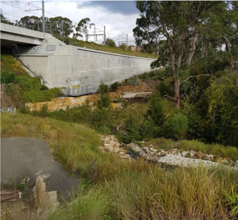
Figure 69 - C2-6 Sediment Retention Basins - Looking South from intersection at M2 exit ramp and Beecroft Road along Devlin's Creek
