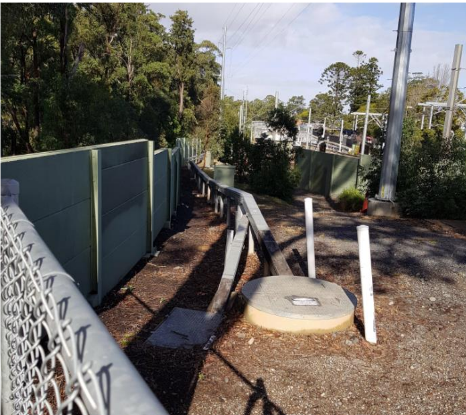
Figure 32 - A2-6 Trees - Looking South along corridor at TfNSW driveway between Chapman Avenue and Beecroft Station
