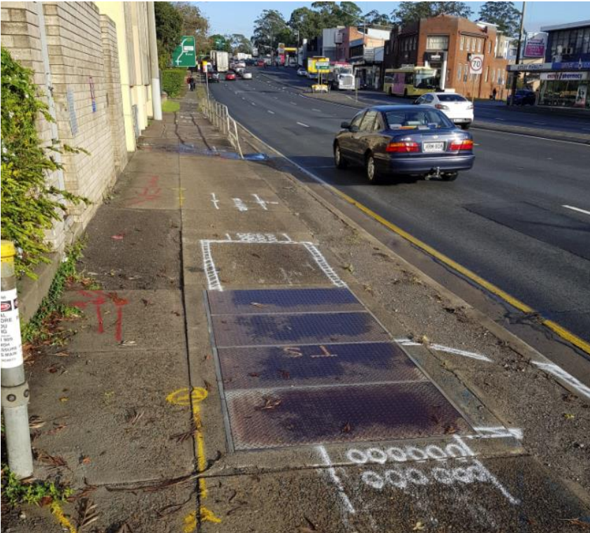
Figure 3 - A1-1 Utilities - Looking west along Pennant Hills Road
