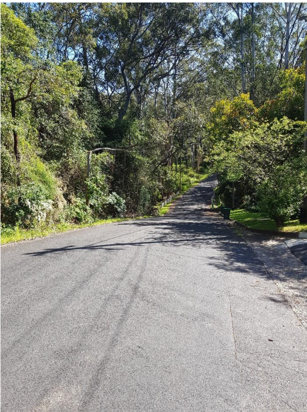
Figure 41 - A4-3 Steep Longitudinal grades - looking north along Sutherland Road towards corner of Sutherland Road and Tristania Way
