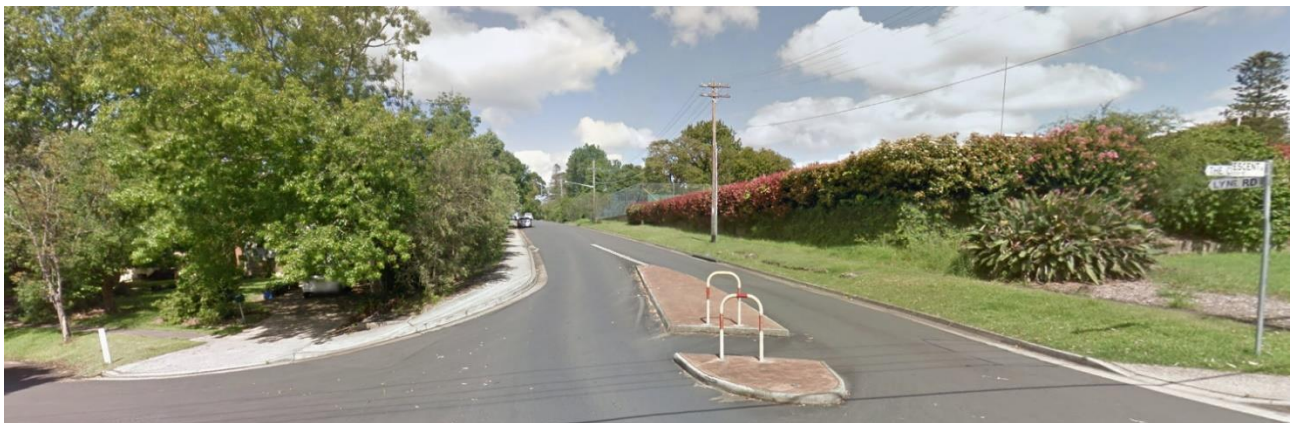
Figure 57 – C1-4 Embankment - Looking South west along Lyne Road [2]
