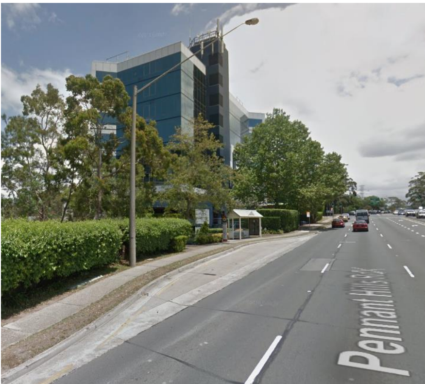
Figure 12 - A1-8 Streetlights/Power Poles - Looking west along Pennant Hills Road [2]
