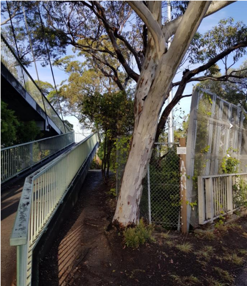
Figure 26 - A2-1 – Narrow Passageway and Tree - Pennant Hills Road looking south west at western side of pedestrian bridge ramp
