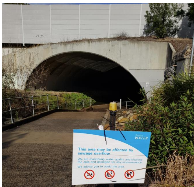
Figure 71 - C3-3 Sewage Overflow and Stormwater- Sutherland Road underpass looking south west.
