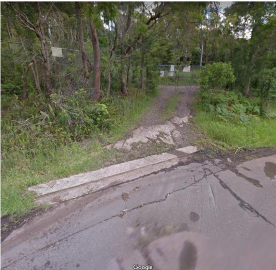
Figure 49 - A4-10 – TfNSW Driveway – Looking north from Sutherland Road (From Google Street View, March 2013 – Accessed 13/12/18)
