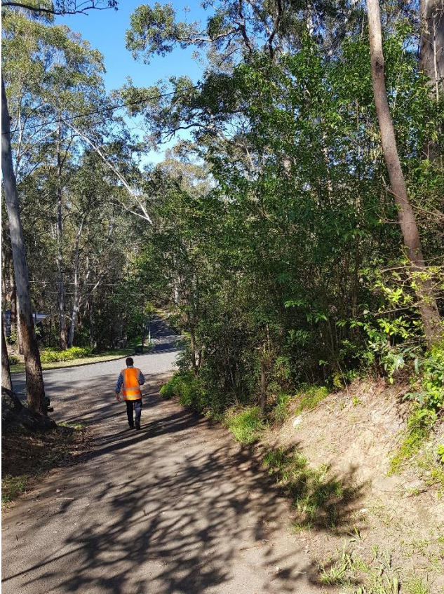
Figure 40 - A4-3 Steep longitude grades – significant longitudinal regrading to provide adequate grades for share path, looking south in the bending along Sutherland Road and Tristania Way
