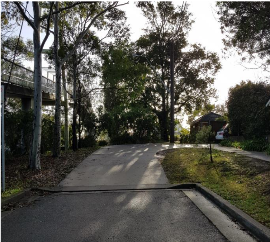
Figure 28 - A2-2 Access Driveway - Hampden road looking north east along eastern side of existing pedestrian overbridge ramp and down local driveway
