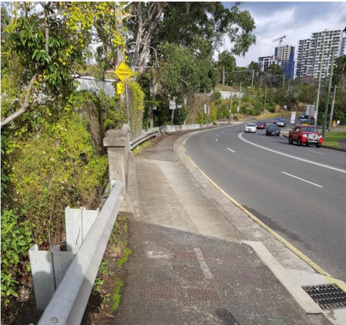
Figure 60 – C1-17 Trees - Looking south along Beecroft Road over Devlin's Creek Bridge
