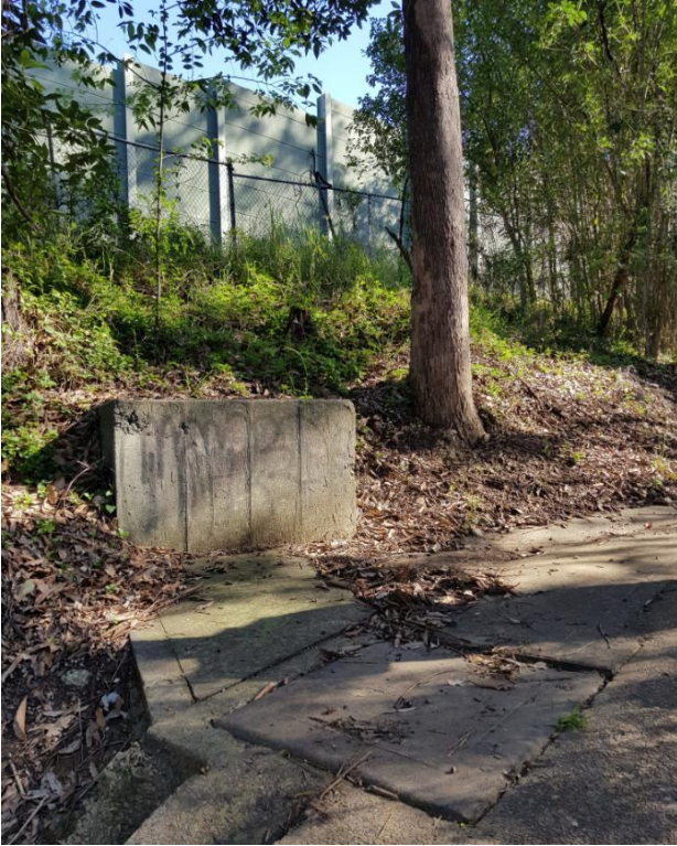
Figure 46 - A4-7 Existing Drainage Pit - Looking north east looking toward the TfNSW maintenance track and noisewall
