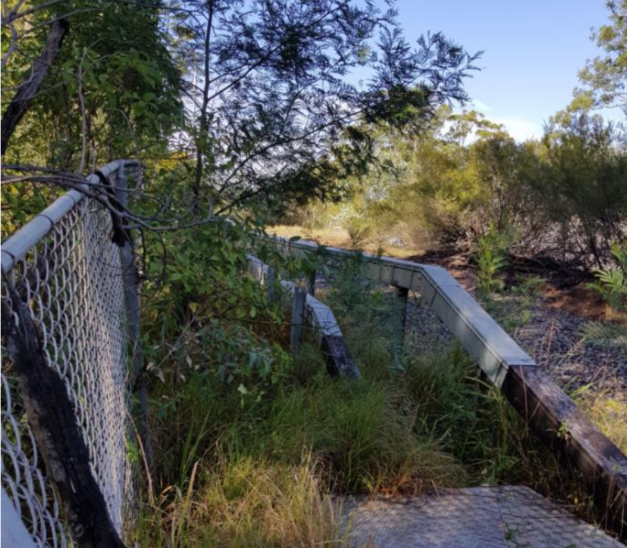
Figure 29 - A2-3 Galvanised steel Troughing (GST) - Looking south along existing maintenance track
