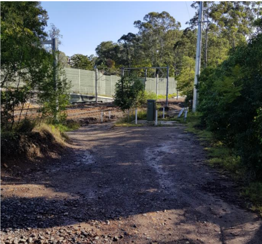
Figure 30 - A2-4 Location Case - Looking north along existing maintenance track
