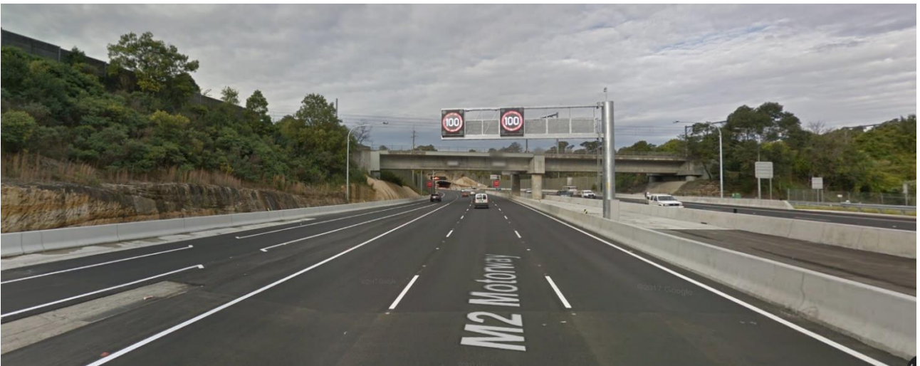
Figure 68 – C2-5 Noisewall, Existing M2 Street lighting and Large Sign Structure - Looking East along M2 showing noisewall, streetlight and large sign structure constraints [2]
