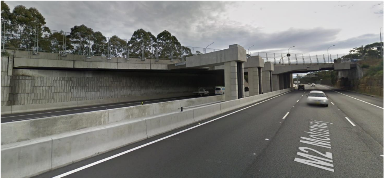
Figure 59 - C1-13 Bridge - Looking East along M2 toward eastern side of Beecroft Road Overbridge [2]
