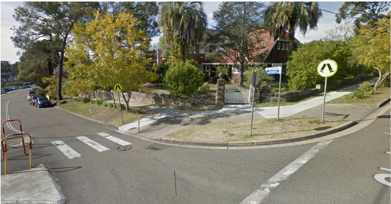
Figure 56 - C1-1 Embankment – Looking south at corner of Cheltenham Road and The Crescent [2]
