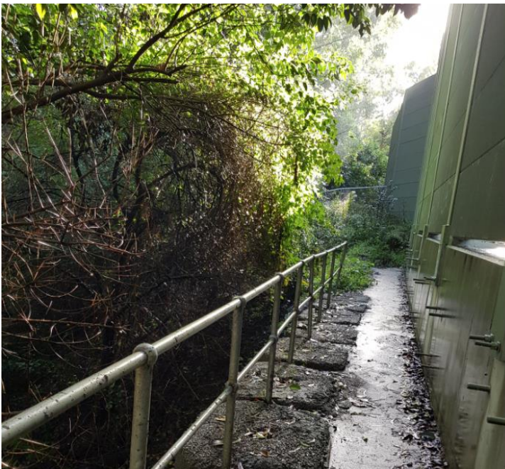
Figure 18 – Byles Creek Crossing - Looking north along existing noise wall
